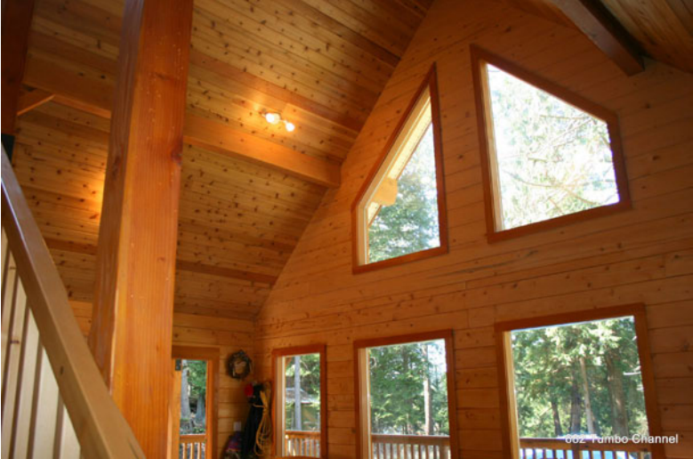
Floor to ceiling red cedar wood finishing
